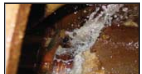
Gland packing 'slime out' consequences
